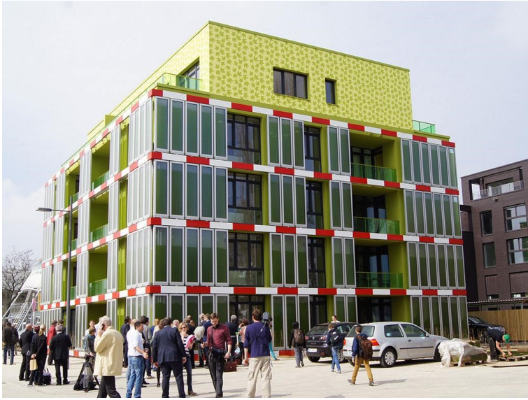
Figure 8: BIQ Hamburg building with algae-facade [19]
