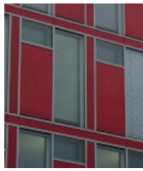
Figure 14: Parapet ventilation at Capricorn Haus [104] [40] (left) and at Siedlungsworks (right) © BINE Informationsdienst FIZ Karlsruhe
