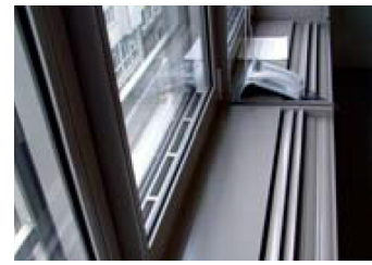
Figure 14: Parapet ventilation at Capricorn Haus [104] [40] (left) and at Siedlungsworks (right) © BINE Informationsdienst FIZ Karlsruhe
